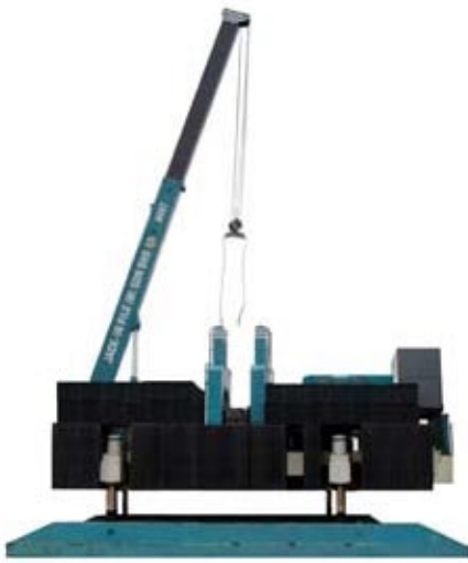
800 tons hydraulic Jack-in machines with crane.
